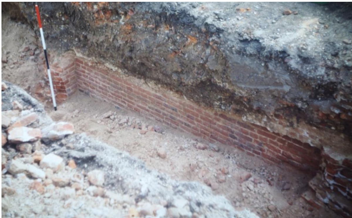
Pl. 5: Walls [152] on the Right, [153] and on the Left the Stub of the Western End Wall of Structure [154] with [153A] above [152] and [153], Looking South.
