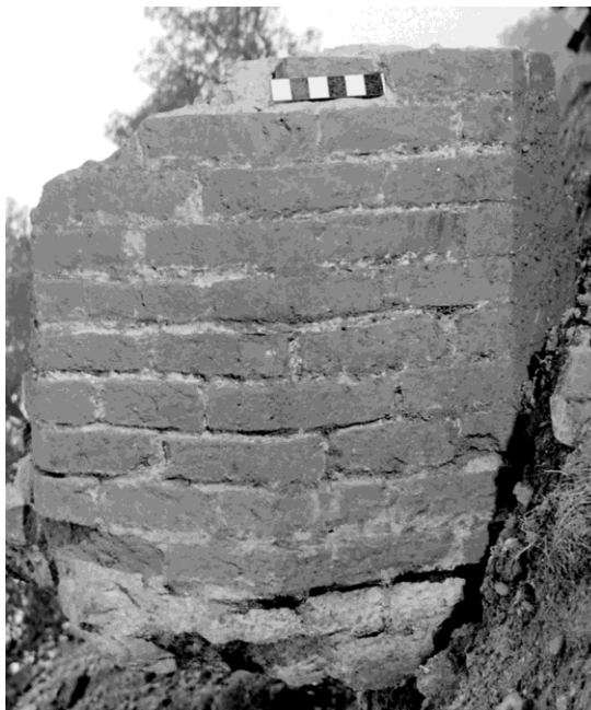
Pl. 13: Octagonal Brick Pillar Contractor Removed from [160].
