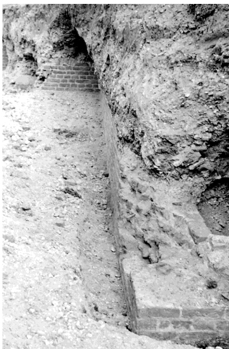
Pl. 3: Wall [150] Looking East.
